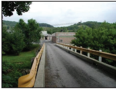
Wastewater Treatment Plant
