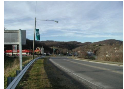
Tazewell Ave. Interchange
